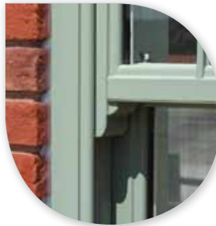
Run through sash horns
